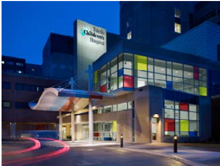
$100 Million Toledo Hospital Renaissance Project 2008 Build Ohio Award Winner Associated General Contractors of Ohio
